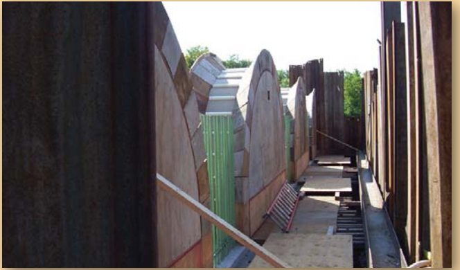
Forming east pier arches
