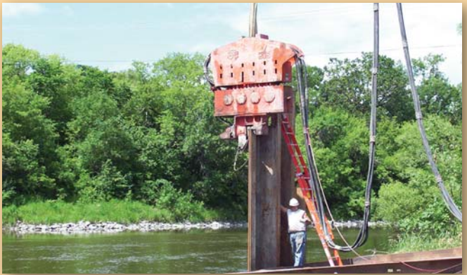
Driving sheet piling for east pier cofferdam
